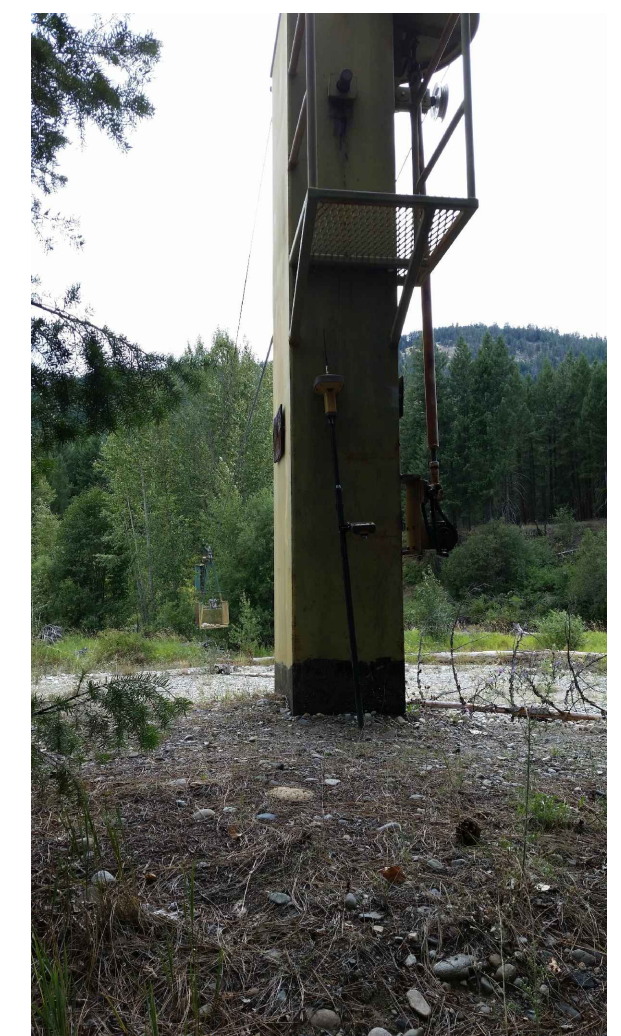
PEOPLE MOVER STRUCTURE AT NORTH SIDE OF RIVER
