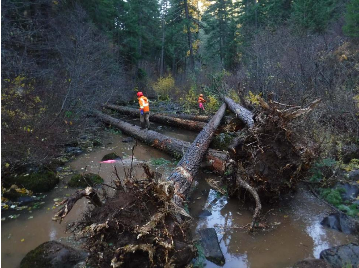
Figure 5. Ground crew removing chokers from helicopter placed logs
