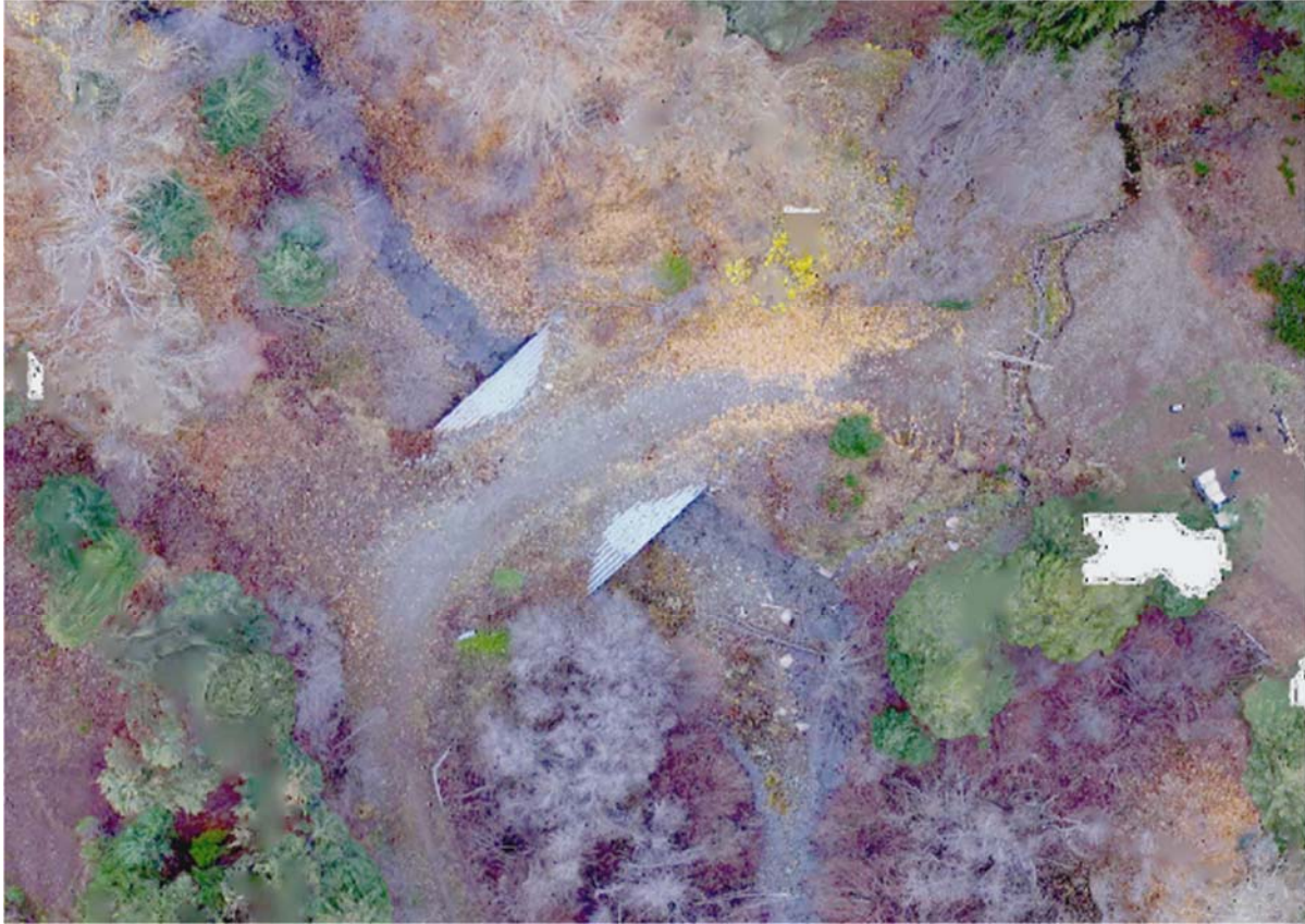
Figure 4. NF-030 Road culvert. Road washout from tributary. From UAV, 2018.
