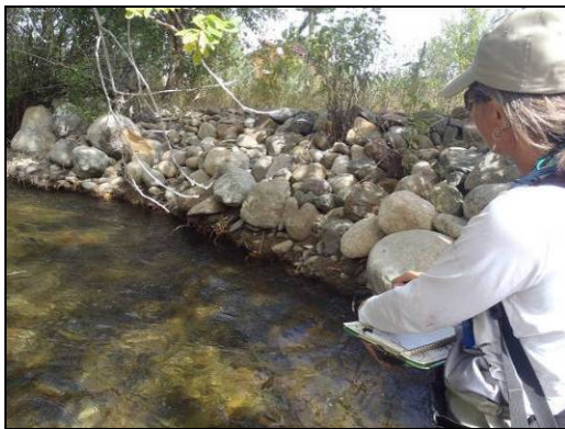
Figure 6. Riprap wall near RM 0.11. The top elevation is approximately 5.5 ft above OWH.
