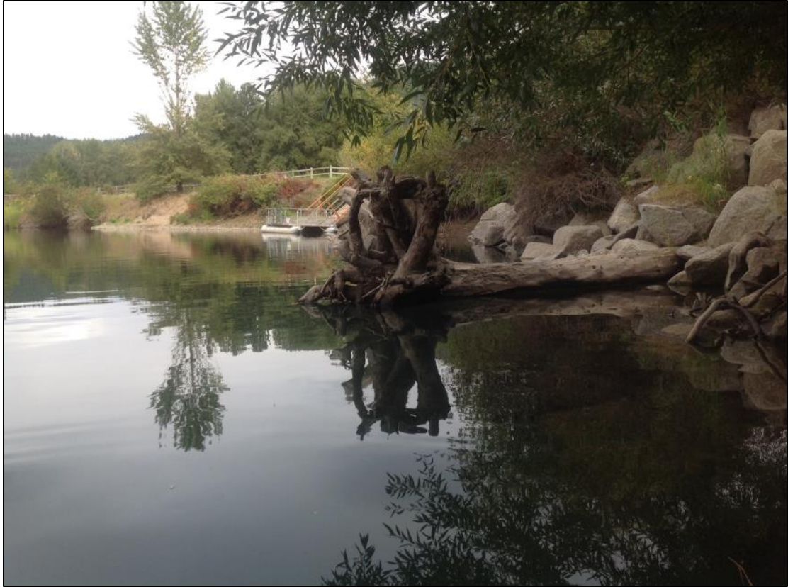
Figure 17. View downstream of single piece of wood with a diameter of 15" and a length of 24' cabled to rip rap along right bank at RM 2.27.
