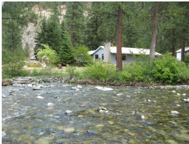
Figure 71. View to the northeast in the downstream direction at the river right floodplain near river mile 5.6. This floodplain area has been cleared and residentially developed. Photo taken in August 2009.
