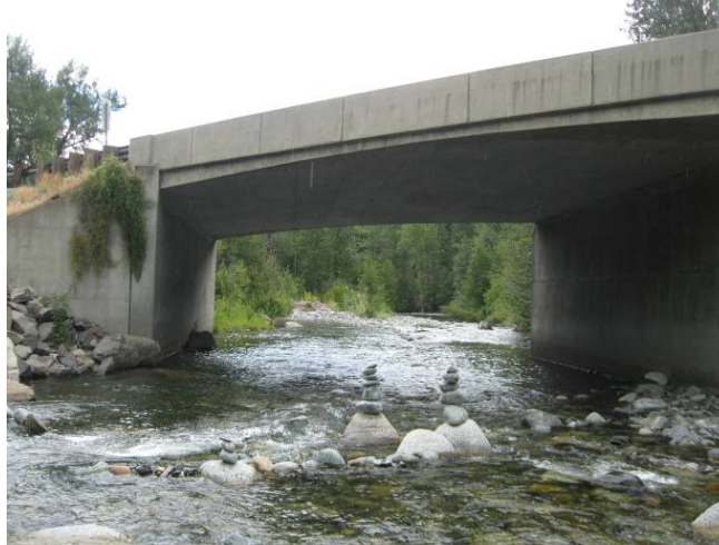
Figure 70. View toward the northeast in the downstream direction near river mile 5.0. The bridge at this location limits local channel dynamics, and floodplain connection downstream. Photo taken in August, 2009.
