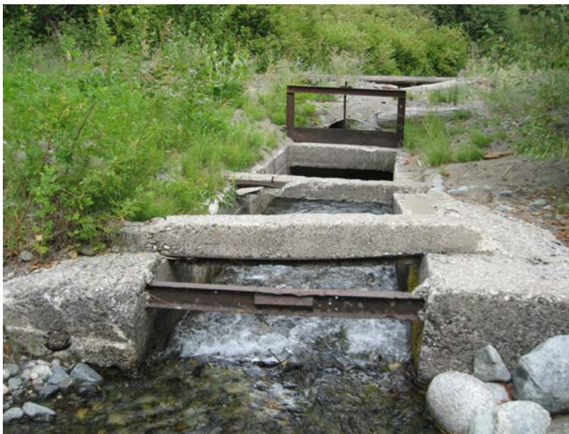
Figure 22. View looking to the north at the Tandy Ditch diversion near river mile 4.9.
