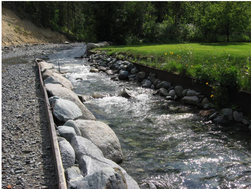
Figure 46. Fish passage channel at diversion dam at river mile 2.5. (August 2009)
