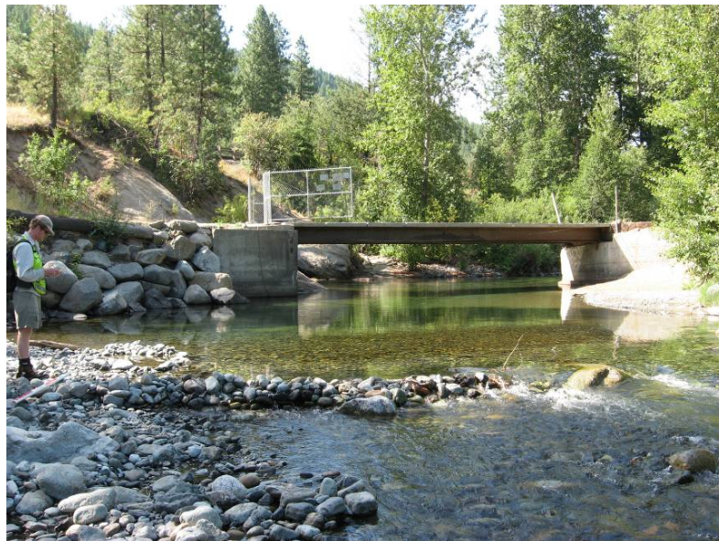
Figure 78. View looking toward the southwest in the upstream direction near river mile 6.45. This narrow private bridge creates hydraulic and geomorphic constraints on the channel and floodplain. Photo taken in August 2009.
