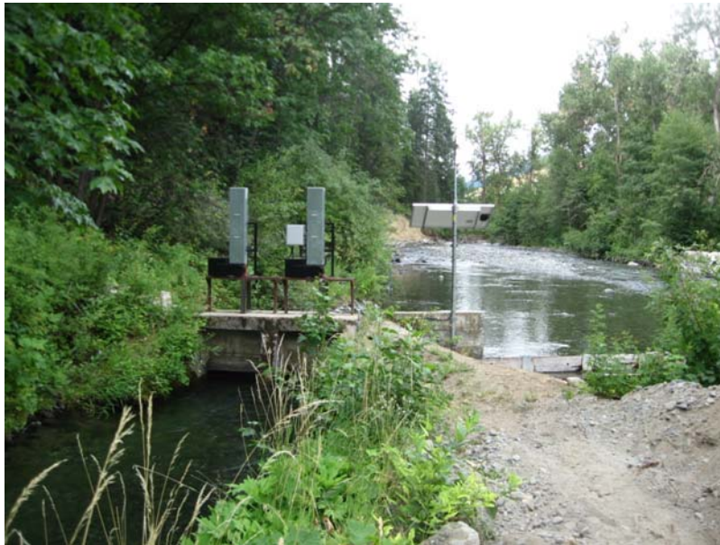
Figure 21. View looking upstream toward the southwest at the Peshastin Canal diversion near river mile 2.5.
