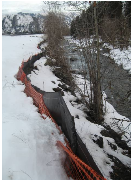
Figure 59. View looking downstream toward the northeast along the former Highway 97 road embankment. Rip-rap was left in place along this channel margin, and enhanced in some locations (January 2010).
