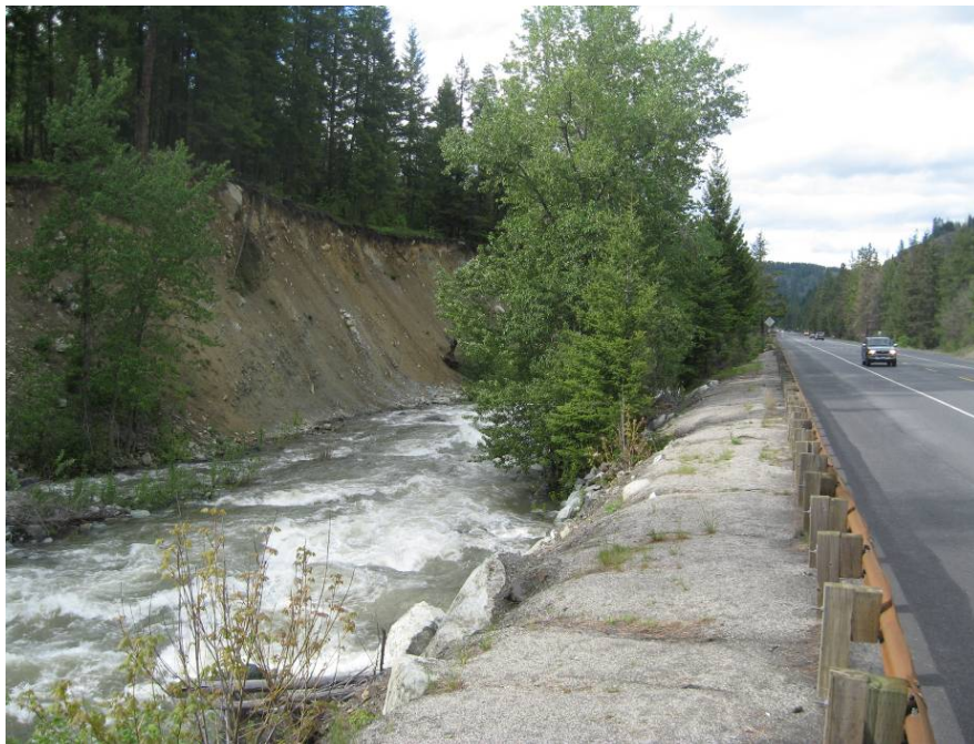
Figure 86. View downstream just downstream of the Ingalls Cr confluence. Hwy 97 directly abuts the channel and contributes to erosion of the high glacial terrace on the opposite bank (May 2010 Photo).
