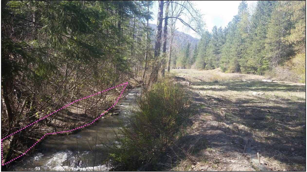
Figure 6. Skinney Creek looking upstream near station 21+00 showing in-set floodplain formation (pink outline) within the steep side slopes. The berm (seen in the center of the image) is relatively short and narrow at the upstream end of the project area.
