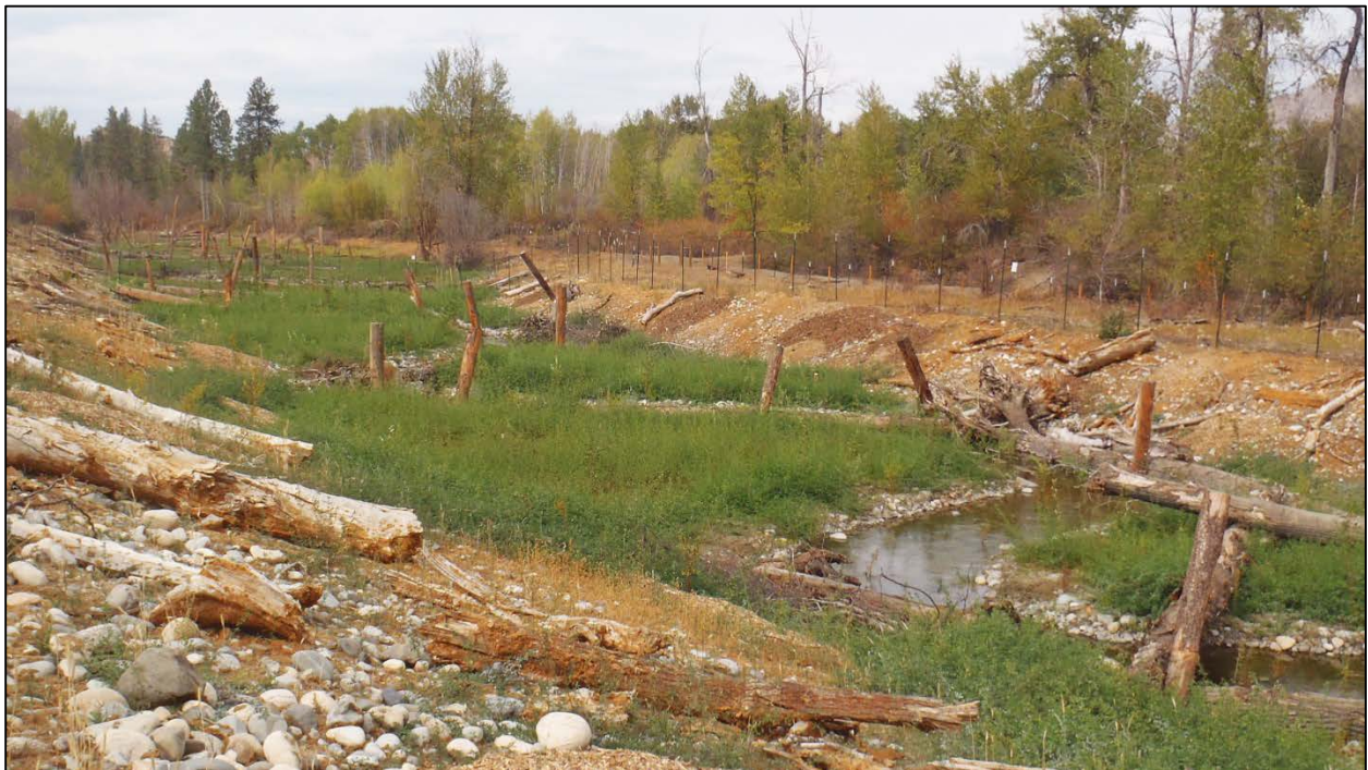
Figure 9. Example of proposed planform showing a meandering channel within a vegetated inset floodplain. Upland species will be planted along slopes to provide shade and future large wood recruitment.
