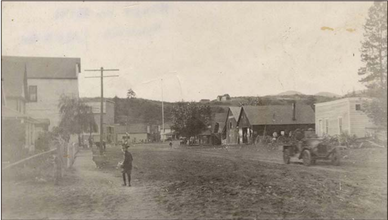
Figure 3. Downtown Winthrop during the early days when the streets were made of dirt. The buildings to the right, including the blacksmith shop, stood where Winthrop Motors and Glassworks now stand. Photo courtesy of the Shafer Museum and the Methow Grist Archive.
