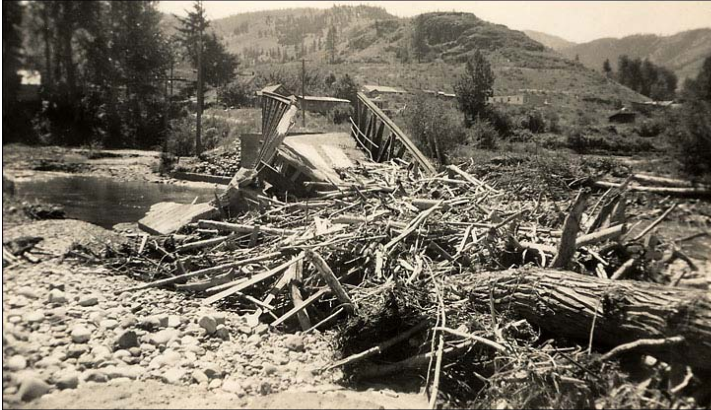
Figure 19. Debris pile and destroyed bridge along the Twisp River by the old creamery after the flood of 1948. Photo from the Wink Byrum Collection, courtesy of the Shafer Museum and the Methow Grist Archive.
