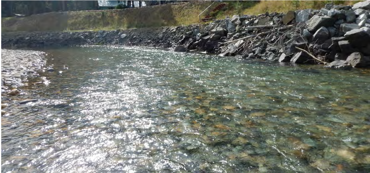
Figure 60. Riprap protected cut bank toe in Reach 3 on river-right at RM 65.30. (9/3/2014)
