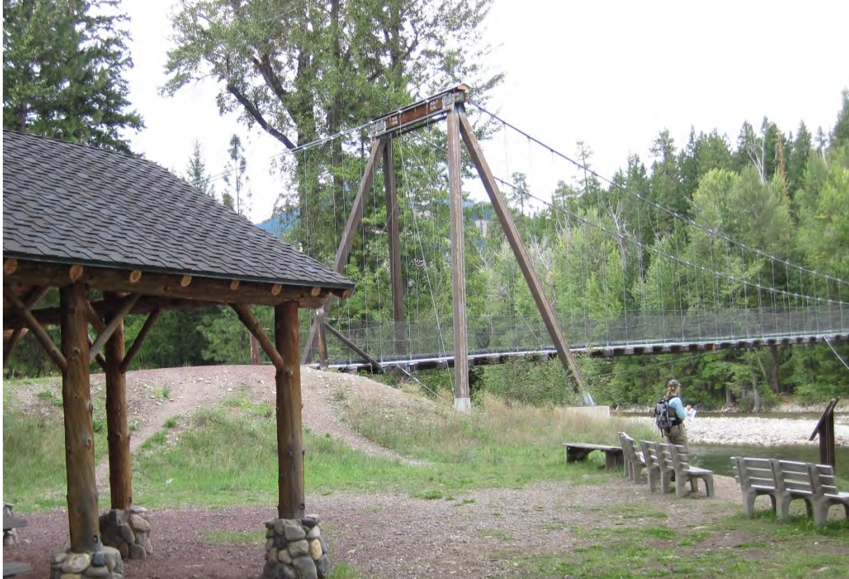
Figure 47. Suspension footbridge abutment and public area on downstream side of bridge on disconnected floodplain at RM 64.35. (9/3/2014)
