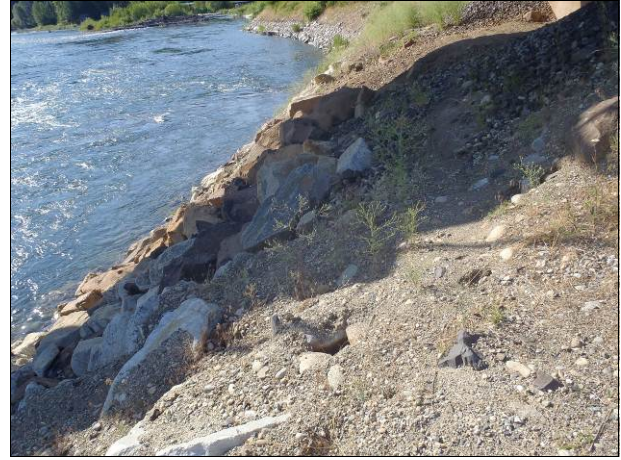
Figure 53. Right bank armoring
