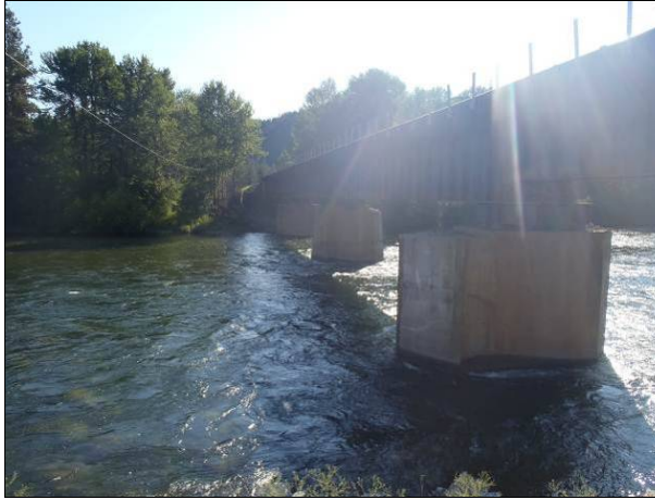
Figure 52. Burlington Northern Railroad Bridge Pilings
