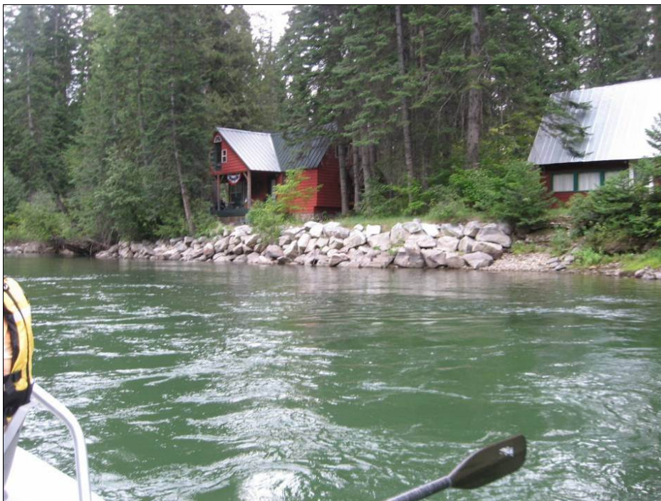
Figure 17. Residential development and bank hardening near the upstream end of the study area.
