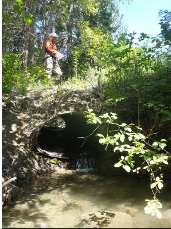
Figure 45. Perched culvert in Deadhorse Creek (RM 38.6). Surface water connection was present on day of survey (July 26, 2011).
