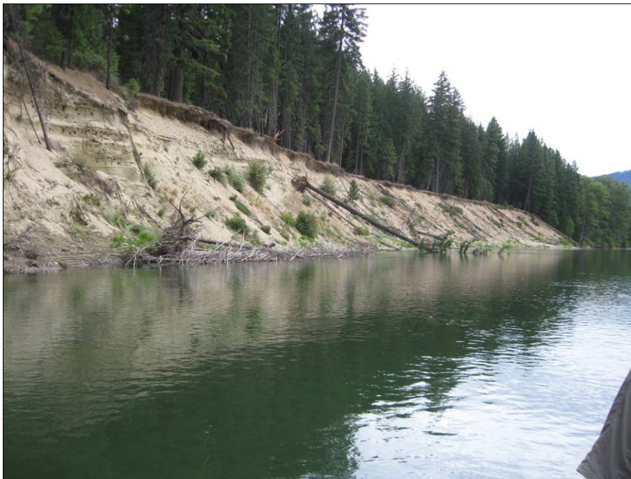
Figure 26. View of unconsolidated fine grain sediment in terrace slopes along the channel in the study area.
