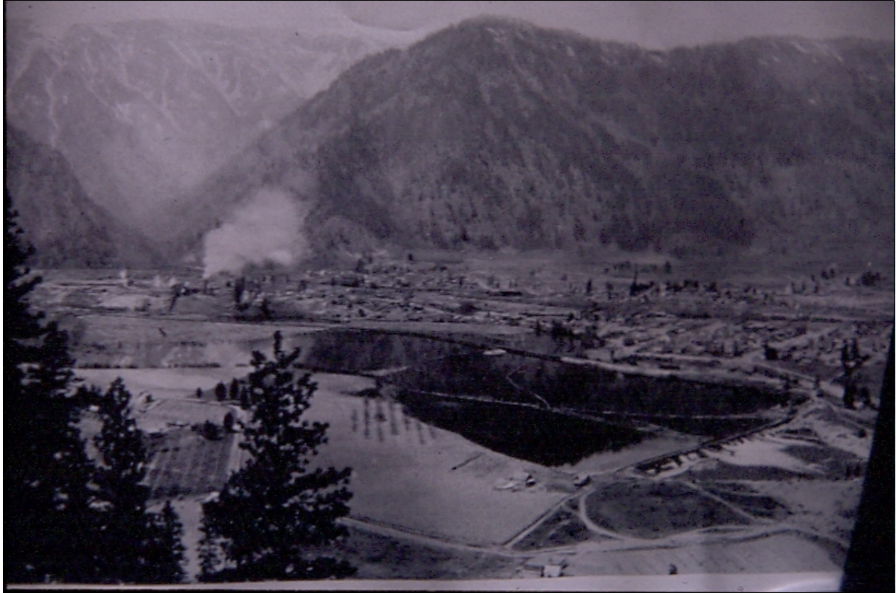
Figure 11. Power dam and mill pond in Leavenworth, WA. Early 1900s.
