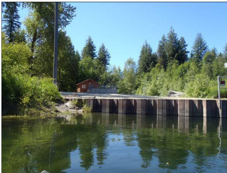
Figure 82. WDFW Chiwawa Ponds Fish Hatchery intake structure.
