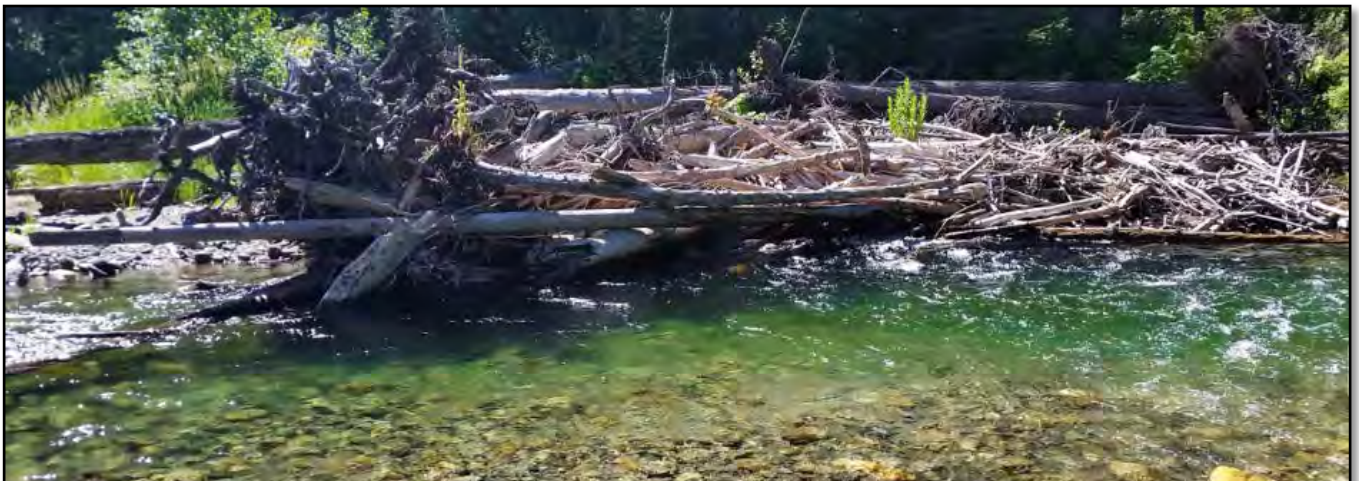
Figure 5: Existing log jam in the S-curve section of the project reach about 1500ft downstream of War Creek Bridge. Flow is from right to left. There are several key-member logs in the 24-30-inch DBH range stabilizing the structure and racking additional material. This structure has completely altered the local planform by forcing a nearly 90-degree turn in the river. A significant scour pool and associated hydraulic/habitat variability is visible in the photo.
