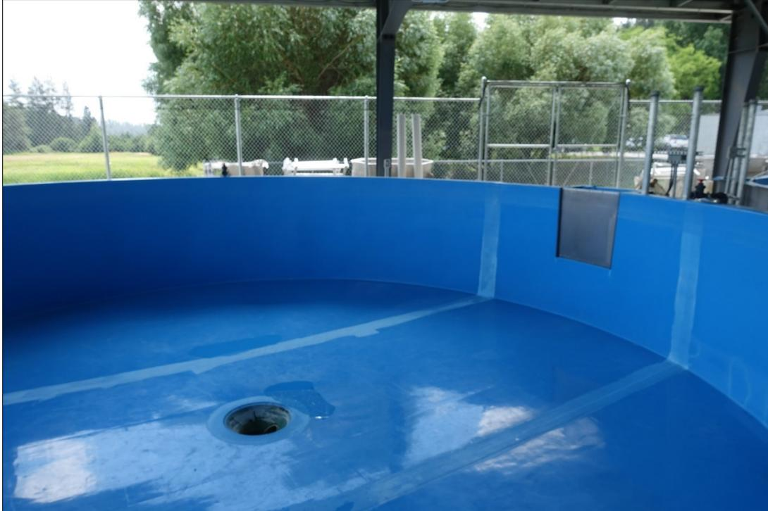
Figure 6-13. 30-Foot-Diameter Circular Tank with Side Drain and Bottom Drain
