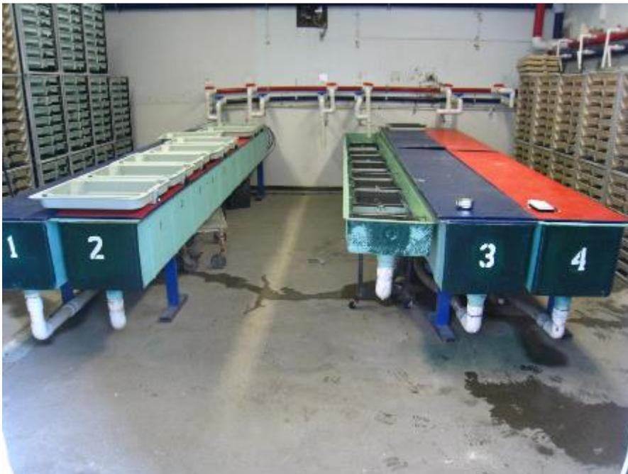
Figure 6-7. Prosser Hatchery incubation room, triple stacks (left), bulk eyeing trough (center) and chilled (blue) and ambient (red) groundwater supply headers
