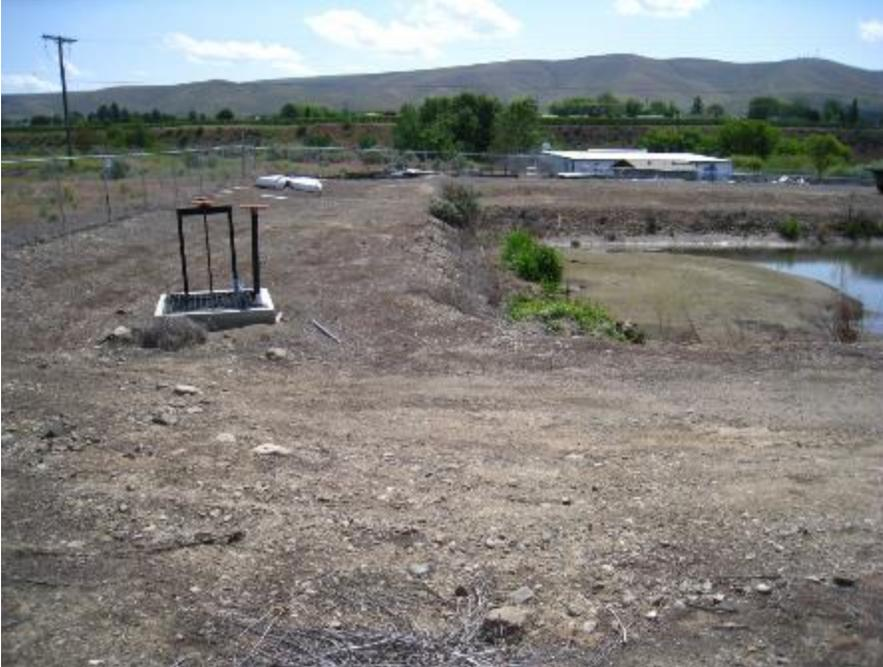
Figure 6-4. River water flow control structure and upper end of silt settling pond at Prosser
