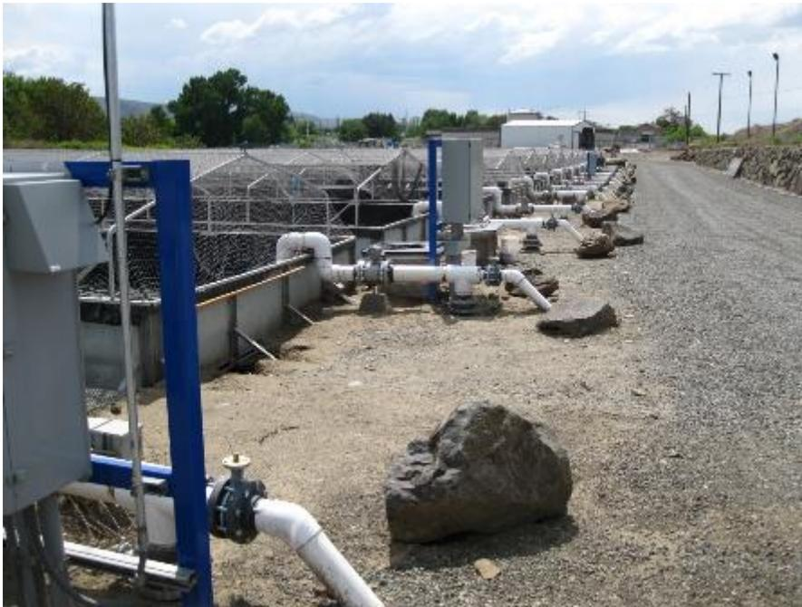
Figure 6-8. Prosser Hatchery dual source process water supply pipes into steel raceways
