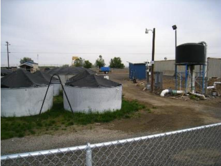
Figure 6-5. Prosser Hatchery Well No. 1 and head box (at right) and steelhead kelt re-conditioning tanks (at left)
