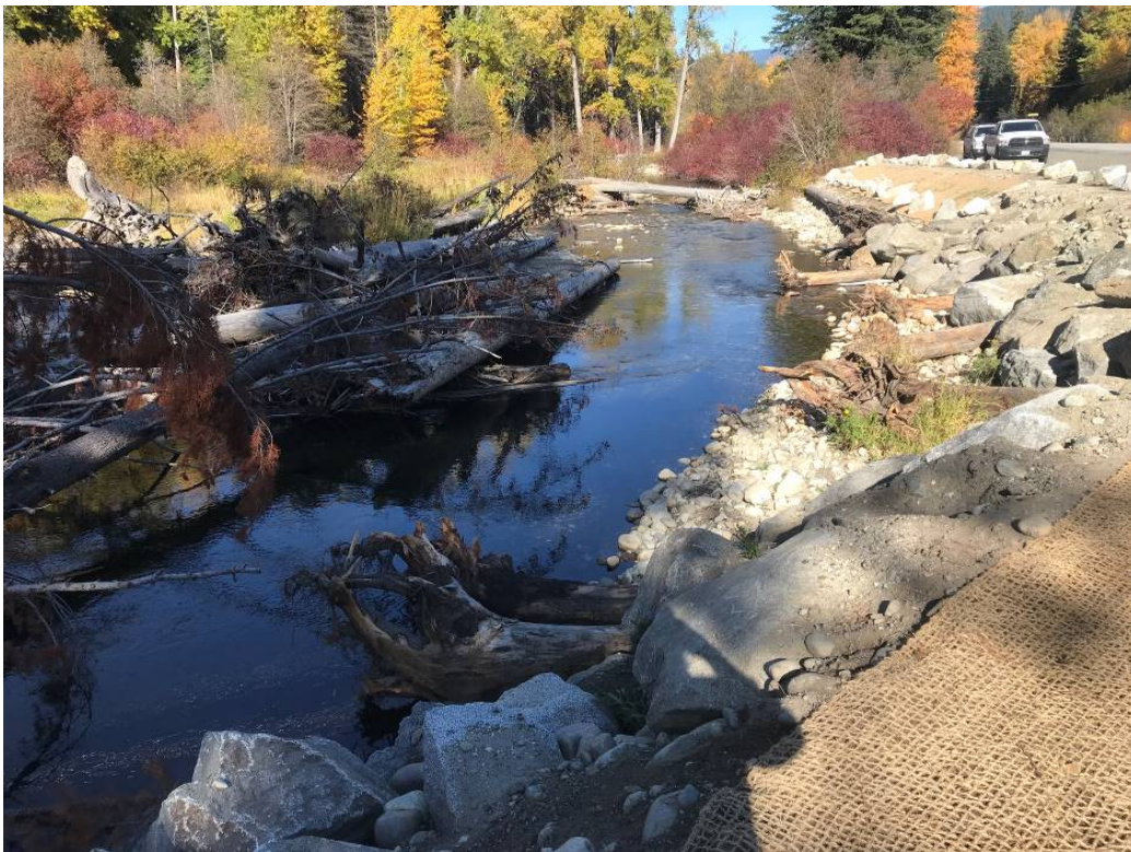
Figure 13. Bank stabilization measures installed in summer of 2018.
