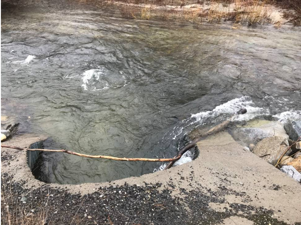
Figure 14. Outlet twelve-foot diameter culvert, installed in 2007.
