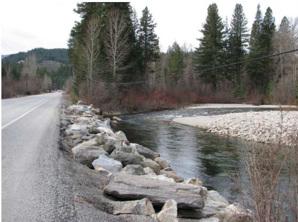
Figure 4. Riprap installed after 1995 flood, from 2010.
