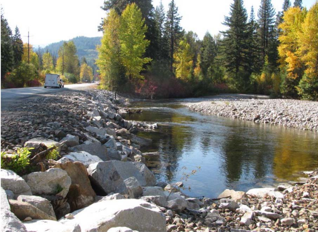
Figure 5. Site conditions in Area 1 in 2011, after addition of rock barbs.
