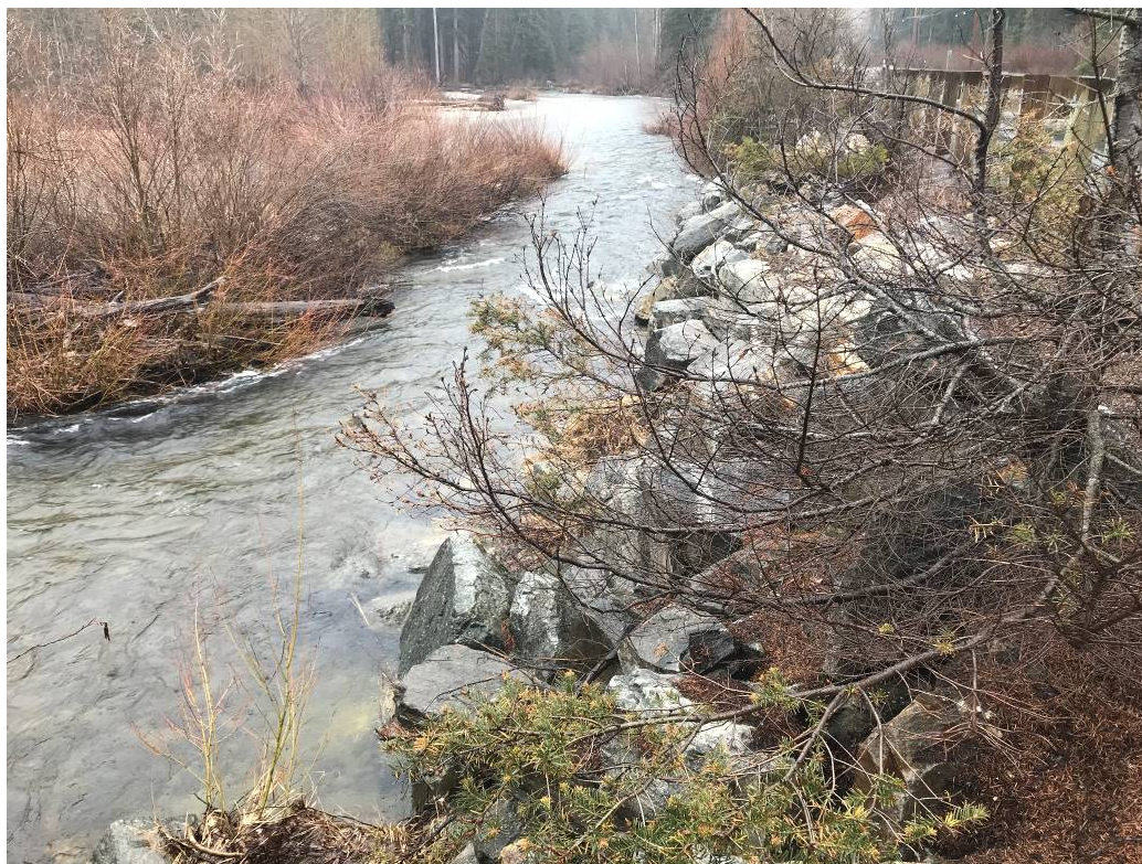
Figure 13. Rock revetment along SR207, April 2018.
