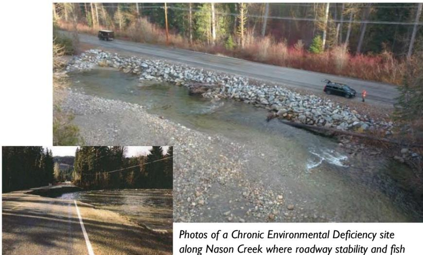
*Photos of a Chronic Environmental Deficiency site along Nason Creek where roadway stability and fish habitat need to be addressed.*
