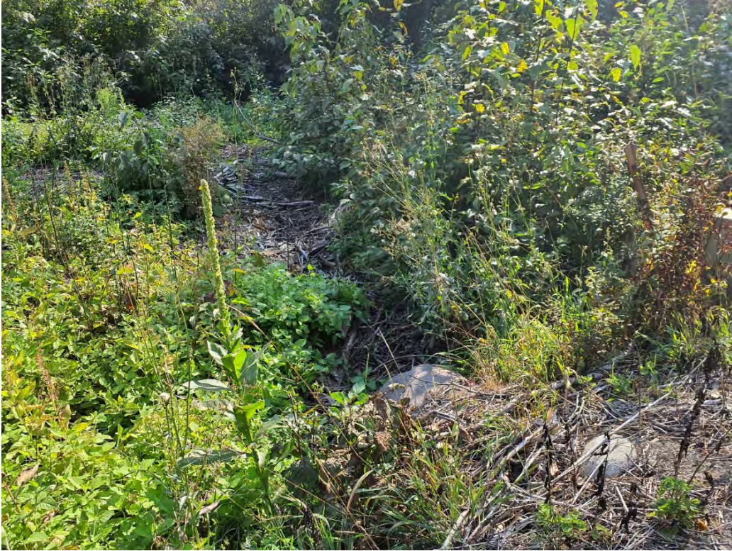
Photopoint 12. Culvert outlet, looking towards WT6. Facing south.
