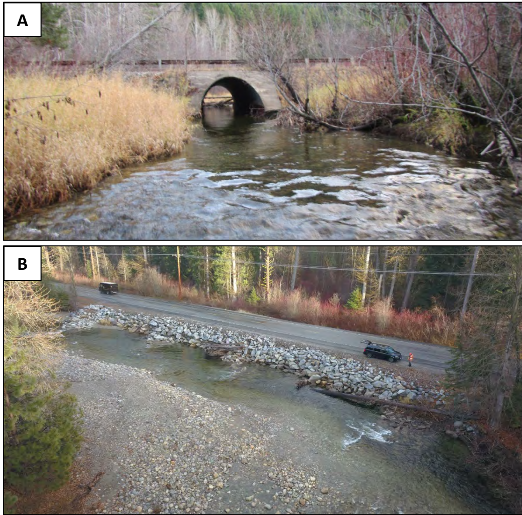
Figure 3. Infrastructure within the project area includes (A) CMP culvert with concrete headwalls (RM 3.75) which provide connectivity to the side channel on the east side of the highway, and (B) Highway 207 (RM 4.4) which has been reinforced with rock in several locations and can be removed with highway relocation and allow hydrologic connection to historic floodplain areas.
