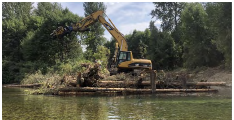
Log structure during construction. (Photo: YN)
