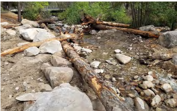
Channel-spanning and habitat forming logs, sourced from adjacent hillslope. (Photos: YN)
