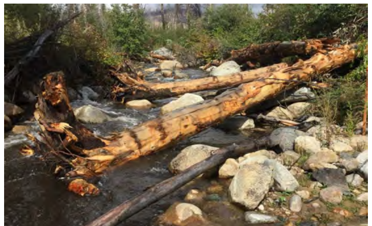
Channel-spanning and habitat forming logs, sourced from adjacent hillslope. (Photos: YN)
