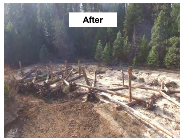
Floodplain reconnected and large wood installed (“after” photo taken before re-watering post-construction). (Photo: YN)
