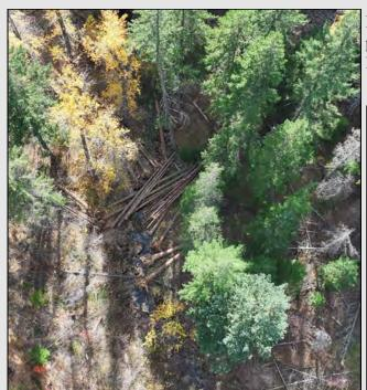
In 2024, we implemented Phase II of the project, during which we placed 267 rootwads, 127 logs, and 174 small wood pieces at 34 log sites over 3.5 miles of White Creek (from river miles 5 to 8).
