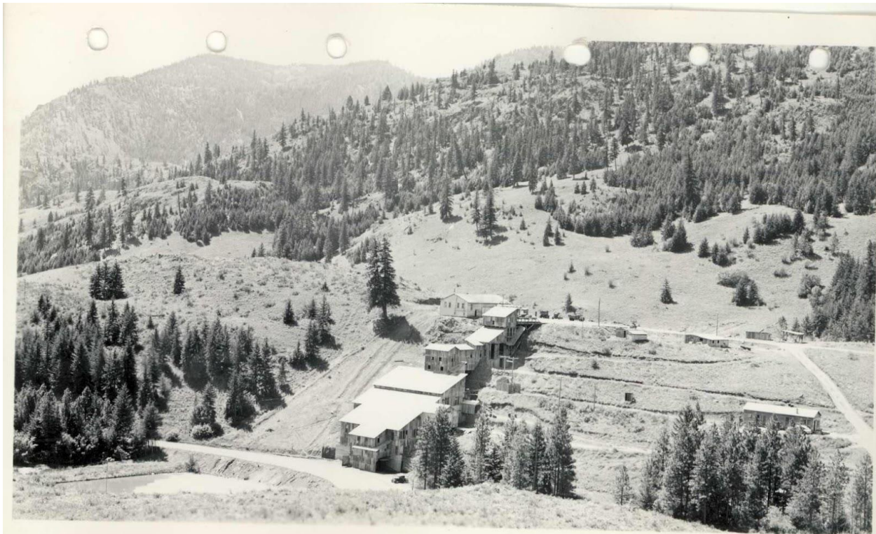
Figure 2. The Alder Mine outside of Twisp (Methow Valley Conservancy 2013).
