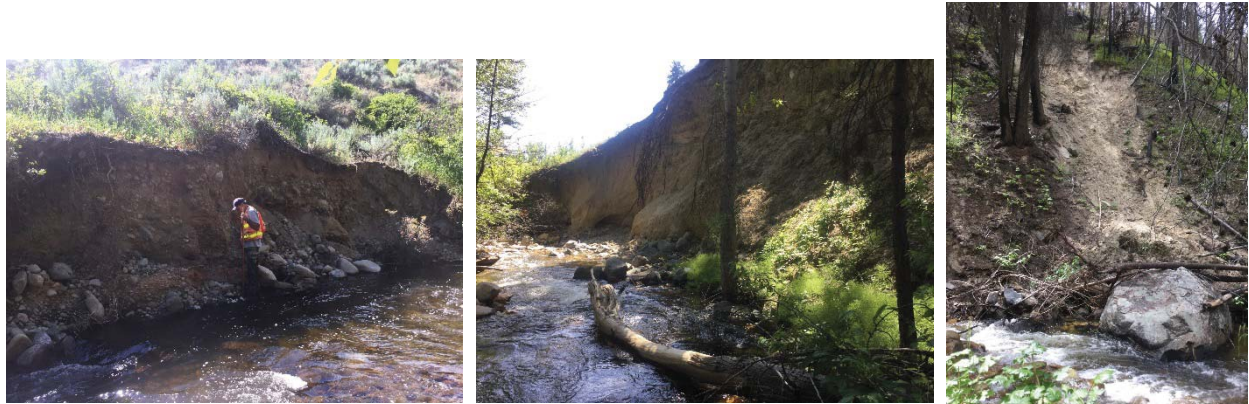
Figure 4-5. Photographs of Typical Eroding Areas Including Bank Erosion near RM 0.6 in Reach 2 (left), Glacial Terrace Erosion near RM 7.9 in Reach 5 (center), and a Stream-adjacent Landslide near RM 10.1 in Reach 6 (right)
