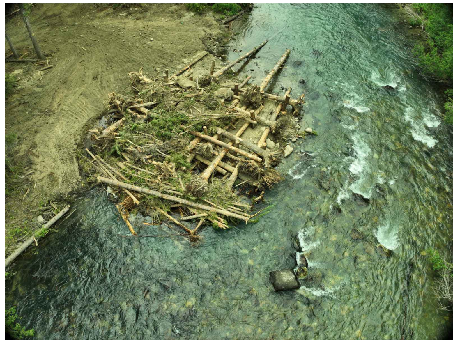
PHASE 1 CONSTRUCTED APEX LARGE WOOD STRUCTURE
