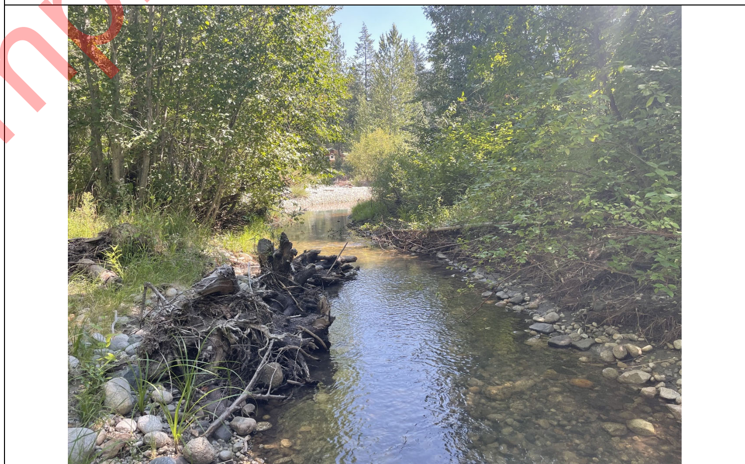
Limited changes in channel geometry since construction in 2021. LWS is intact.
