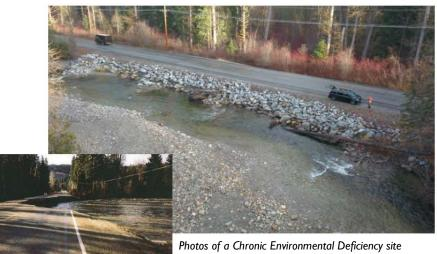
Photos of a Chronic Environmental Deficiency site along Nason Creek where roadway stability and fish habitat need to be addressed.
