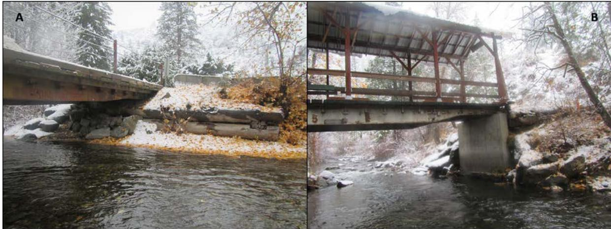
**Figure 30. Railroad-car bridge crossings: A) near RM 0.3 with log, cement, and riprap footings and bank protection. Logs are old footings from historical bridge crossing, and B) near RM 0.6 with cement footings and large boulder riprap. (Photos: 11/9/2017).**
