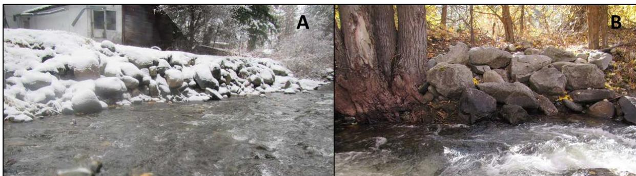
**Figure 31. Riprapped banks: A) river left at RM 0.51 (11/9/2017), and B) river left at RM 0.28 (10/24/2017).**
