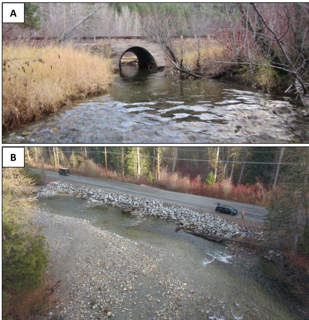
Figure 3. Infrastructure within the project area includes (A) CMP culvert with concrete headwalls (RM 3.75) which provide connectivity to the side channel on the east side of the highway, and (B) Highway 207 (RM 4.4) which has been reinforced with rock in several locations.
