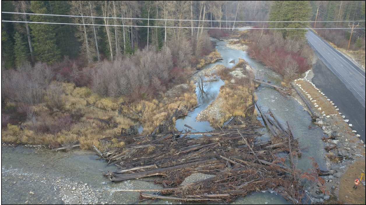
Figure 2. Looking downstream at existing log structure, BPA powerlines, and Highway 207 near RM 4.1.
