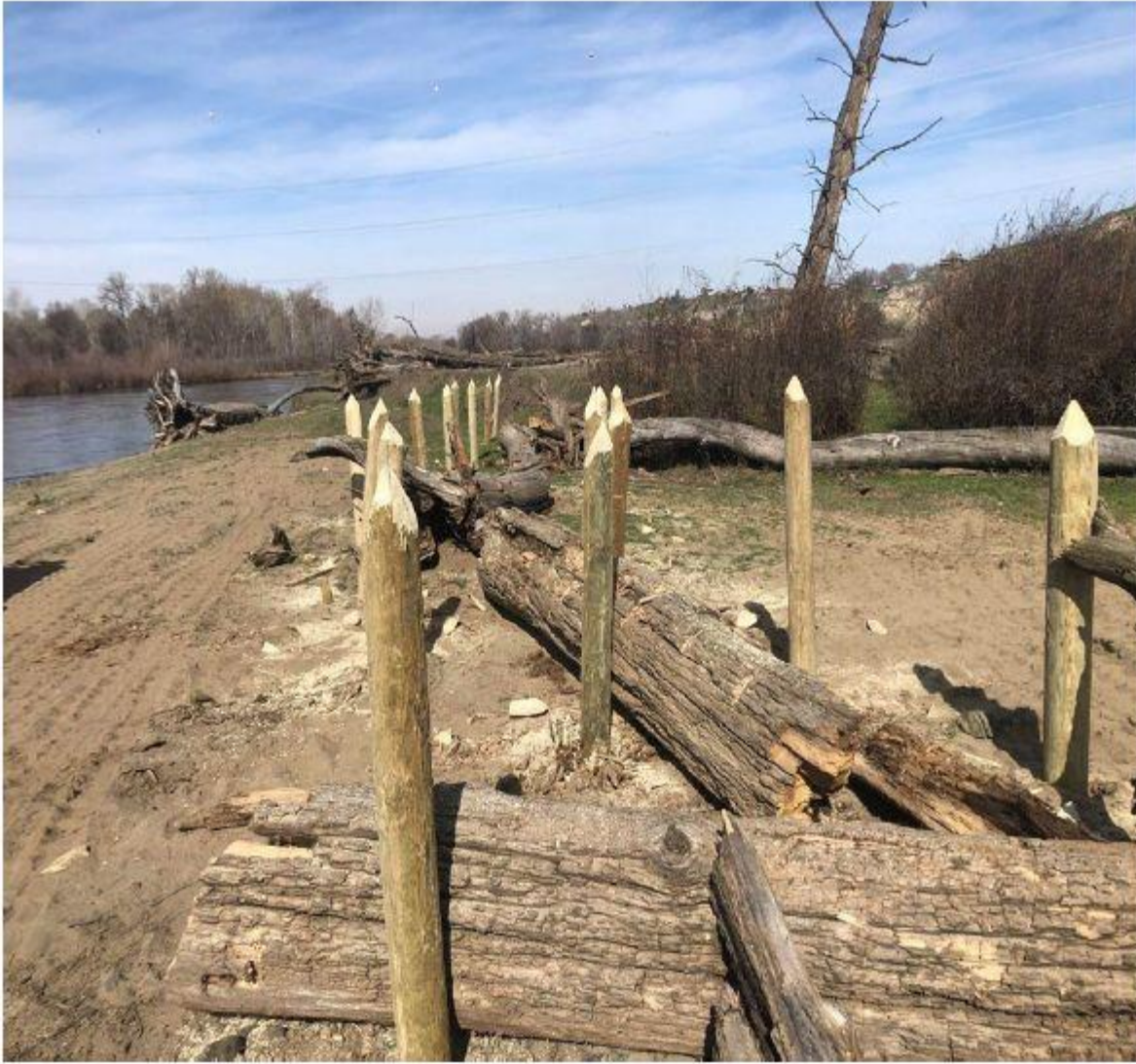
Figure 7. Driven post protection structure 15 miles downstream of the Pond 5 project site on the Yakima River. These structures used onsite woody debris rather than imported logs. Posts are sharpened Per WDFW requirement to deter perching by predatory birds.
