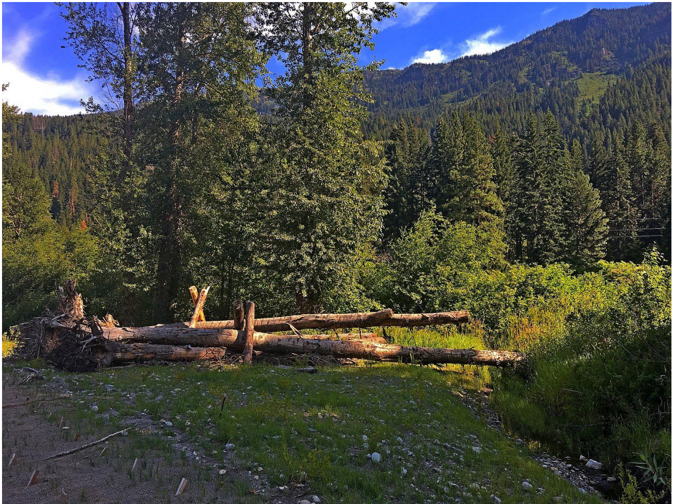
Figure 6. Examples of protective hydraulic structures similar to what is expected at the Pond 5 site. They consist of large logs pinned in place by piles driven in at an angle, to prevent floating. The piles can be driven by hand held pneumatic hammers or by drivers mounted on heavy equipment.
