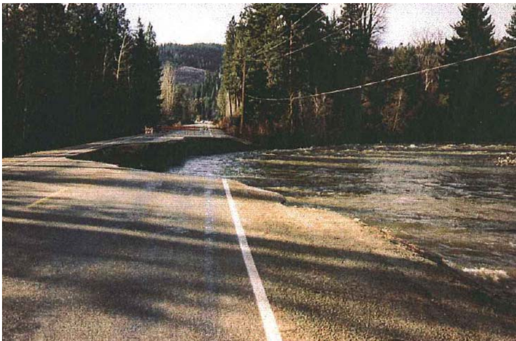
Figure 1 - 1995 flood erosion of SR207 near RM 4.5 (WSDOT photo)
