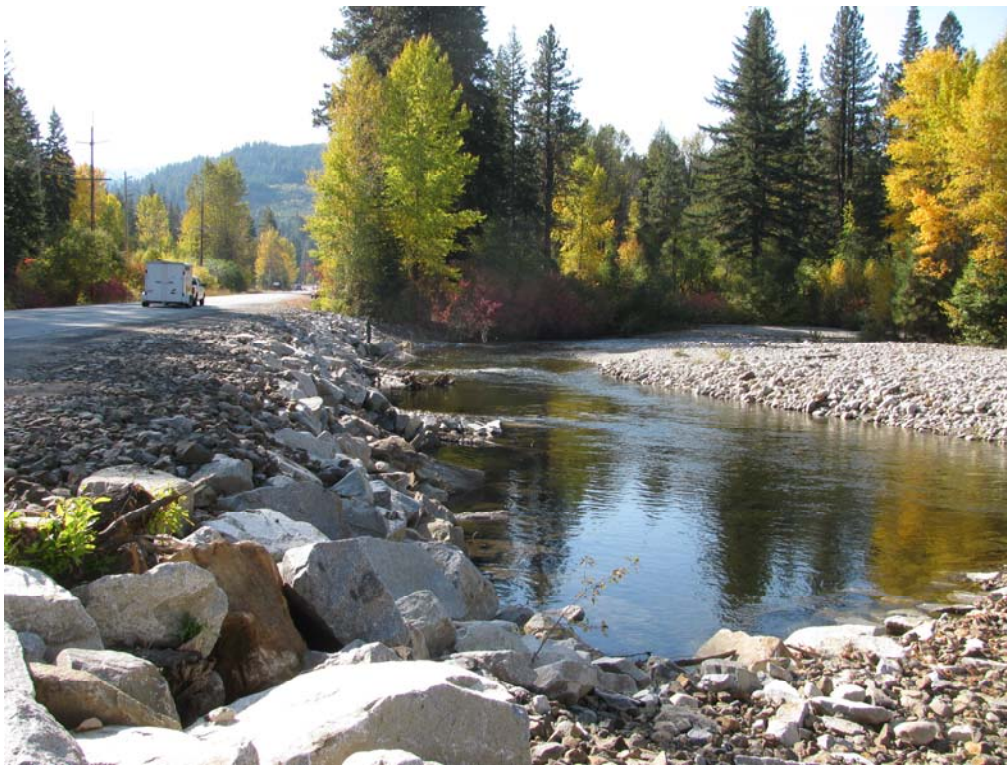
Photo 4: Fall 2011 site conditions in Nason Creek depicting the additional rip rap and rock barbs installed to protect the road prism.
