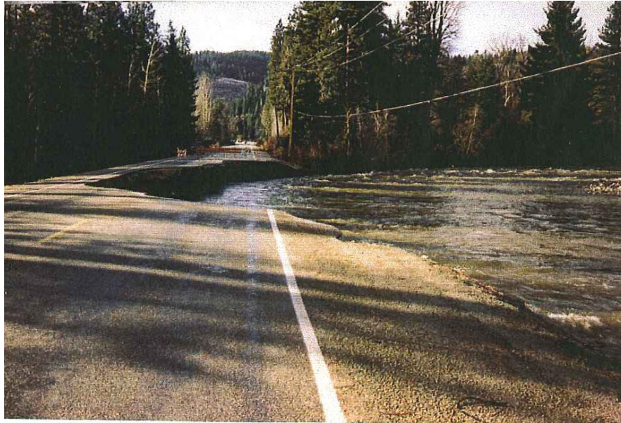
Photo 1: 1995 flood that washed out the SR 207 road prism near RM 4.5. Photo taken from the north looking south.
