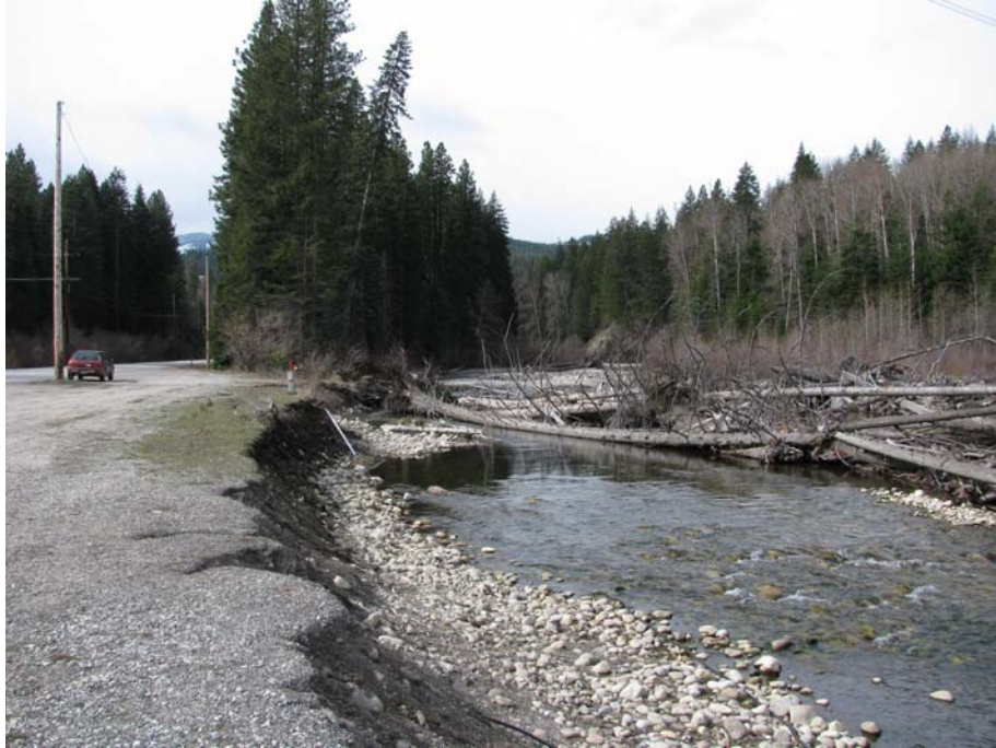
Photo 5: April 2010 site conditions in Nason Creek under the powerline crossing. Note the powerpole and car and distance from the eroding edge of the creek.
