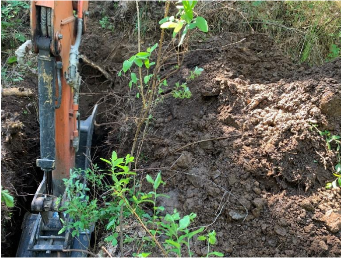
TP-1, Excavating below groundwater, cobbly, wet.
