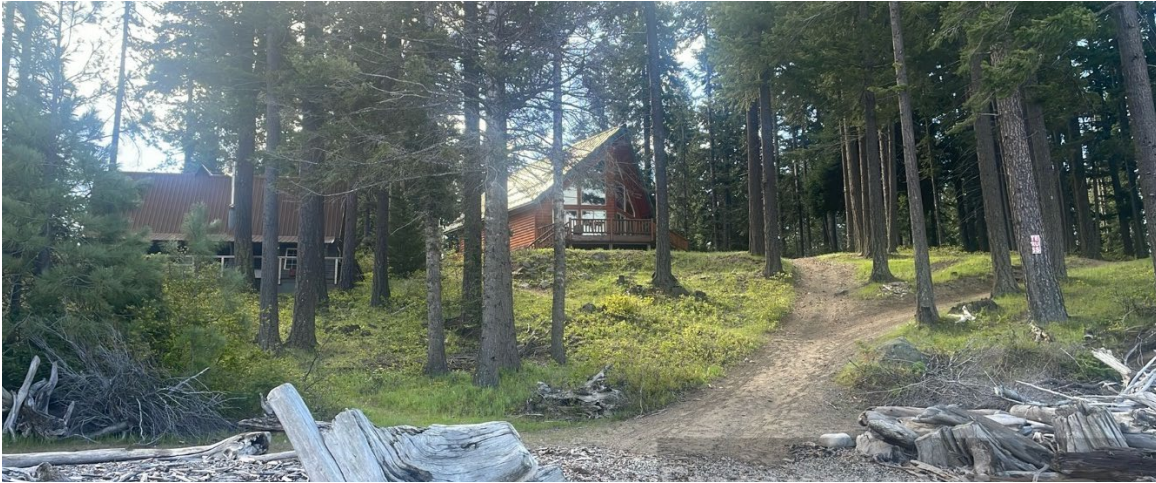
Site Photo 3: Shows typical conditions and trees to be removed along the edge of the reservoir.
