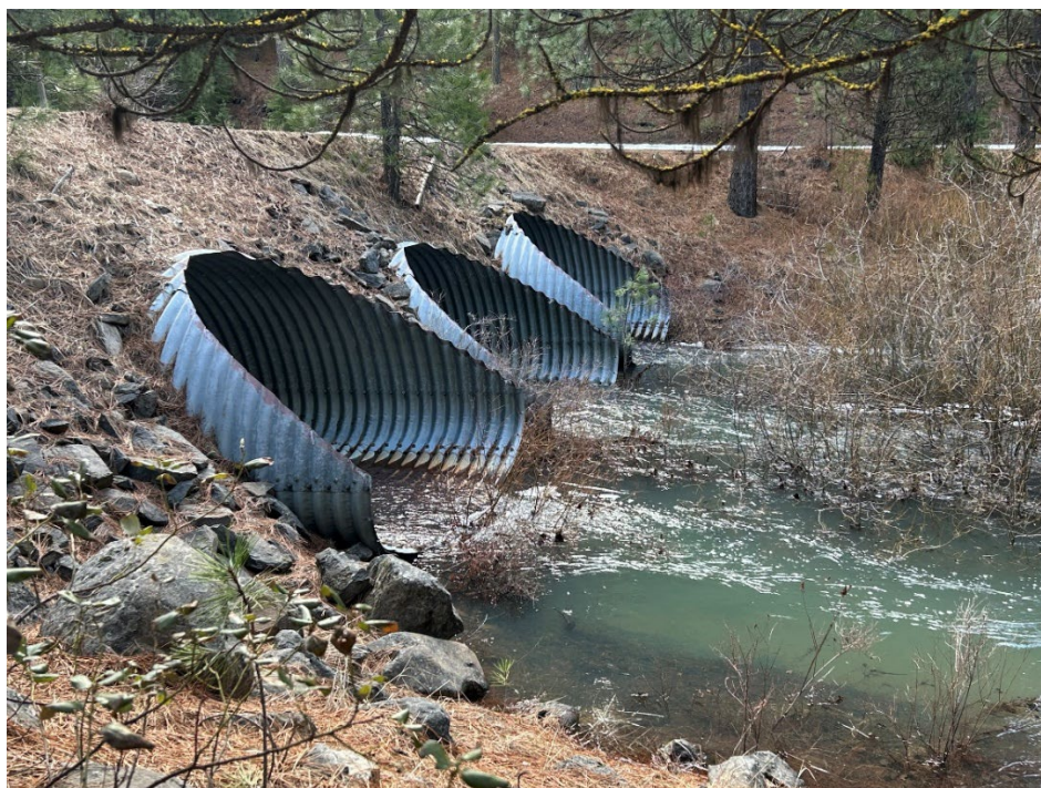
Site Photo 1: Three culverts to be removed, view from upstream side.
