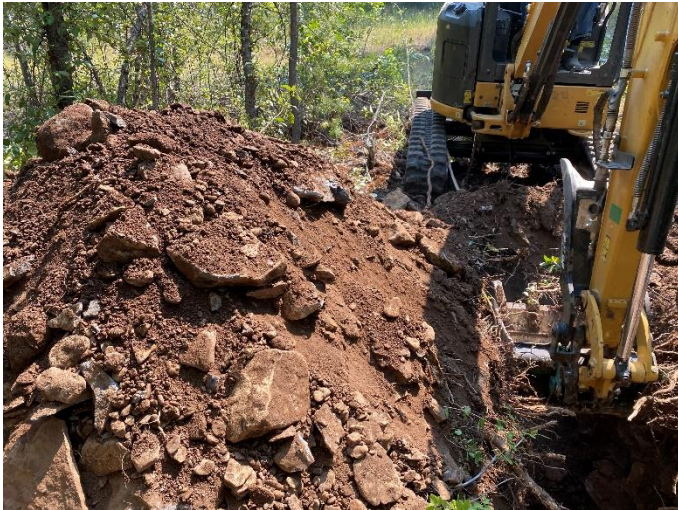
TP-2, stockpile with cobbles and boulders
