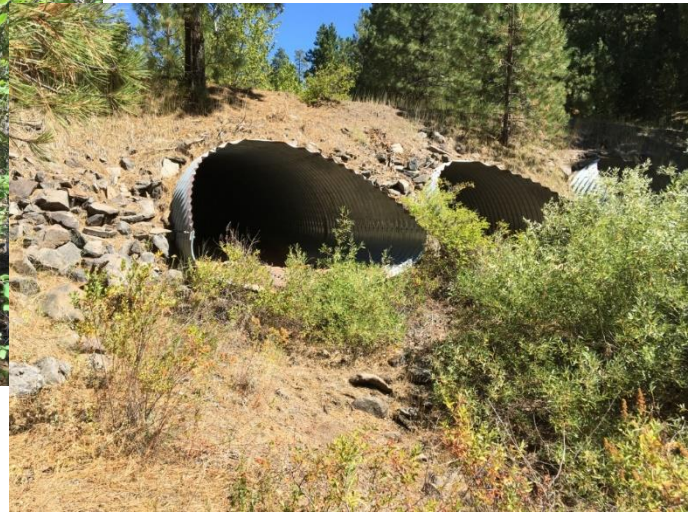
Downstream, looking east
