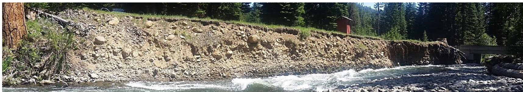
Figure 8. Actively eroding face of left bank approximately 200 l.f. upstream of bridge.
