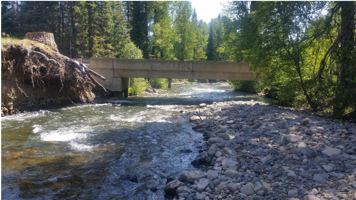
Figure 5. Downstream view of bar accretion (river-right) associated with asymmetrical flow distribution at bridge section.
