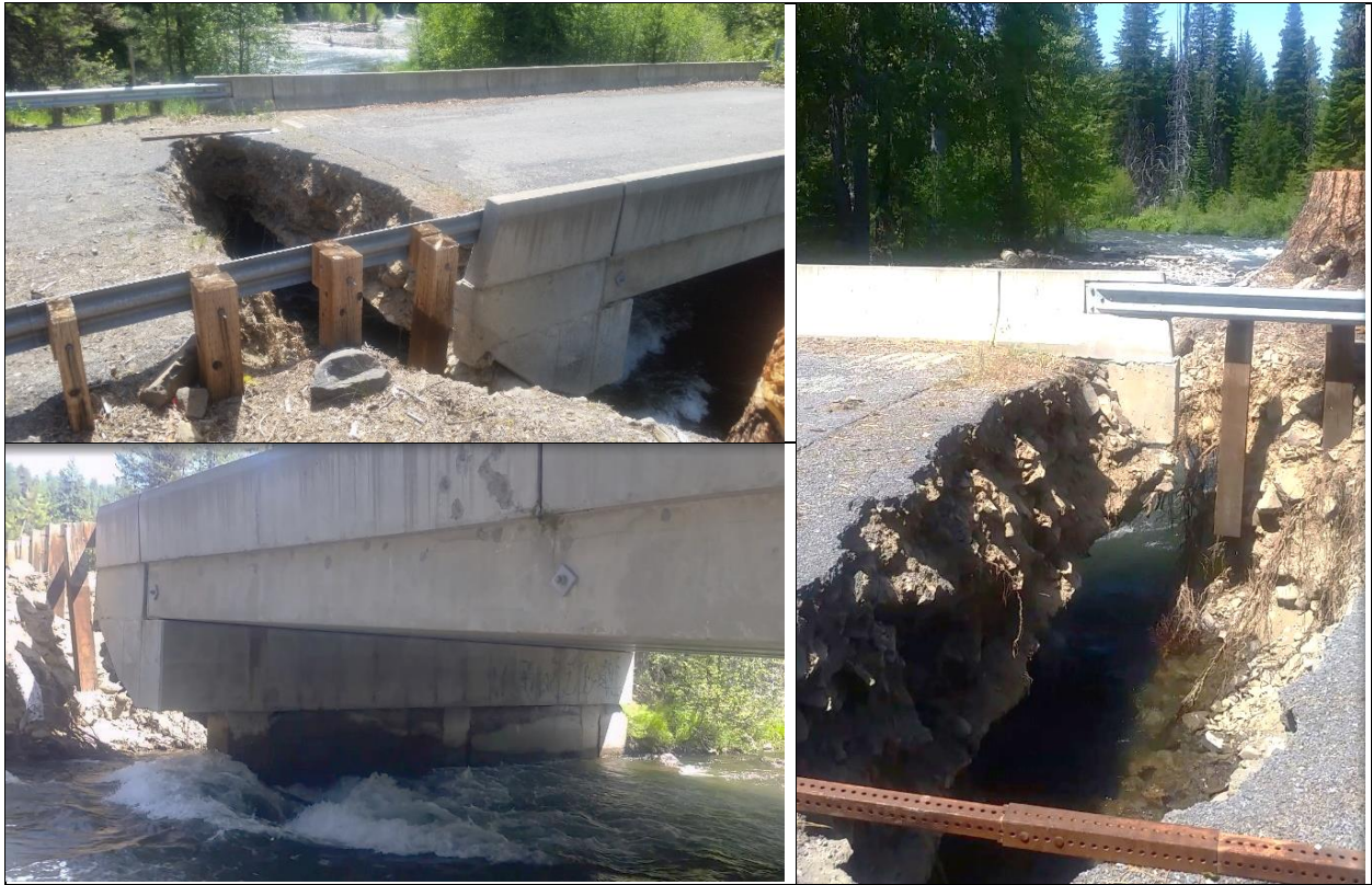
Figure 2. Close-up photos of east abutment washout (all photos taken 6/7/16).
