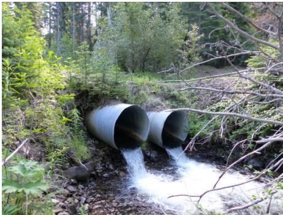
Figure 3. Piscoe Creek 80 Road Crossing current undersized culverts.
