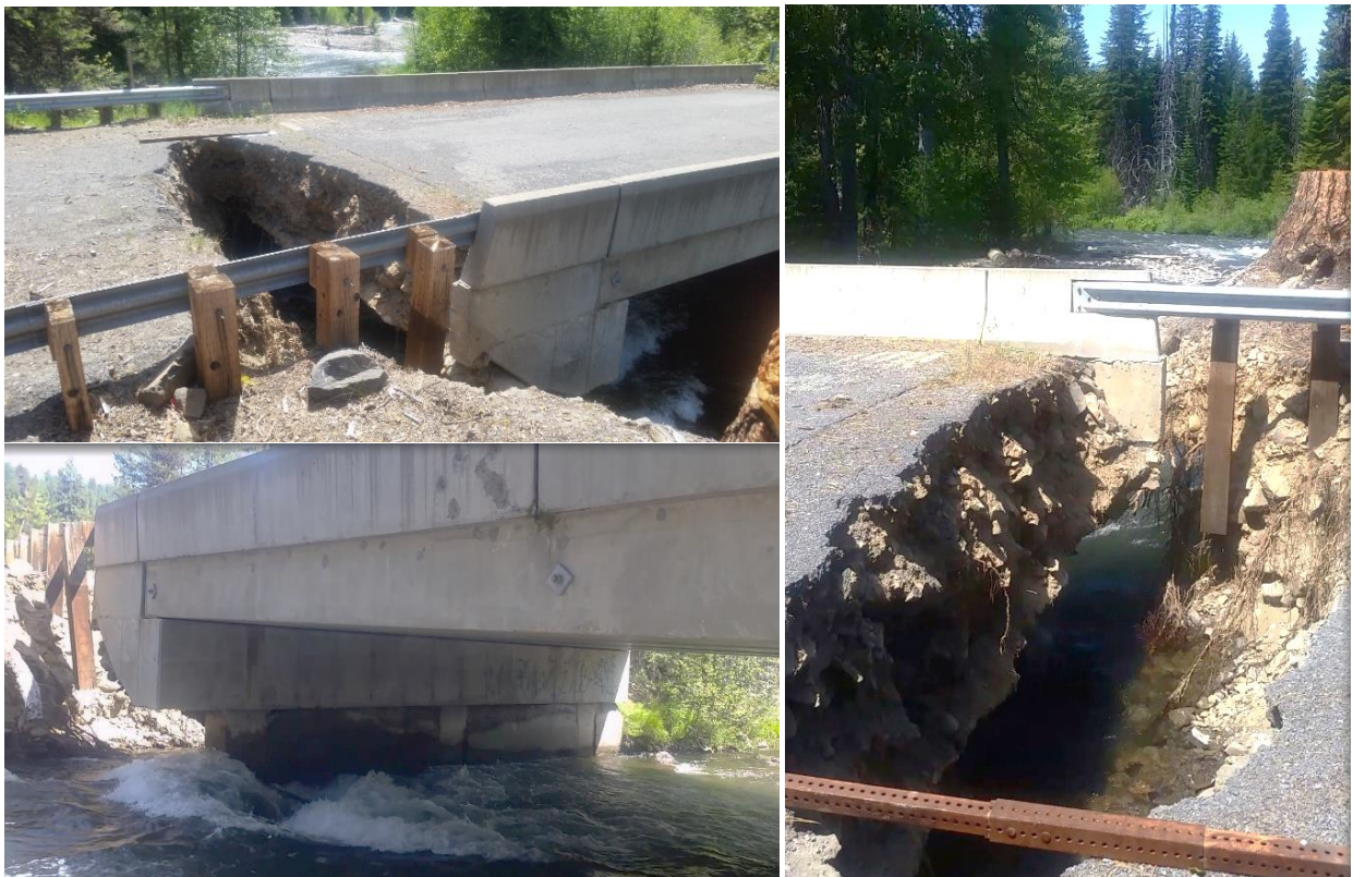
Figure 6. Close up photos of east abutment washout (taken 6/17/2016).
