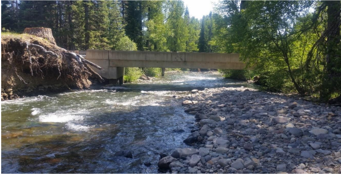
Figure 5. Downstream view of bar accretion (river right) associated with flow distribution at the bridge.
