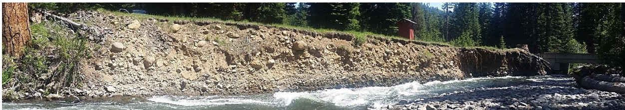
Figure 7. Actively eroding face of left bank approximately 200 l.f. upstream of bridge.
