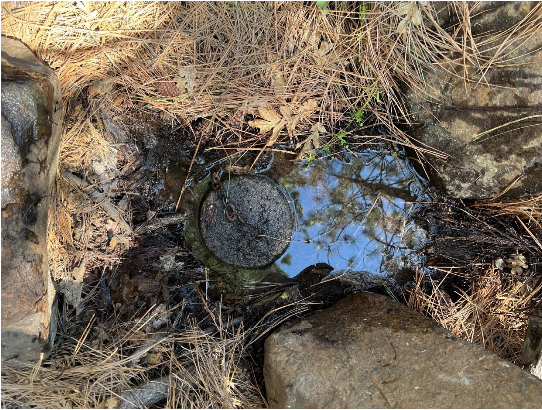
Figure 5. Existing spring box at Worksite #1.
