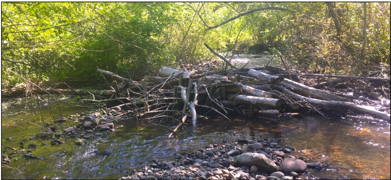
Figure 10. Example of a mid-channel post-assisted log structure (PALS) designed to mimic woody debris accumulations.
