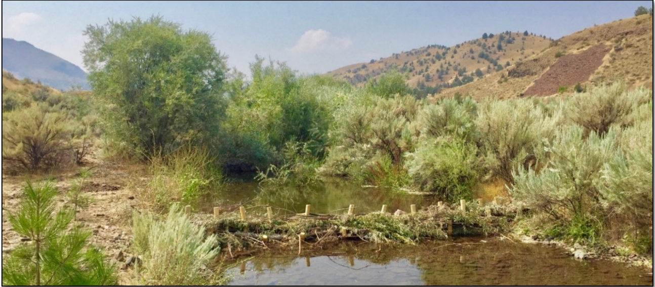
Figure 11. Example of beaver dam analogue (BDA) reinforced with posts.
